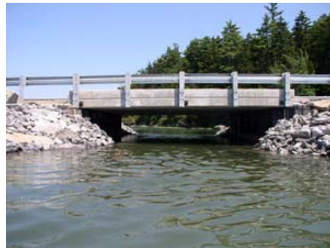
Figure 2: New Dingley Island Bridge After July 2003 Construction
